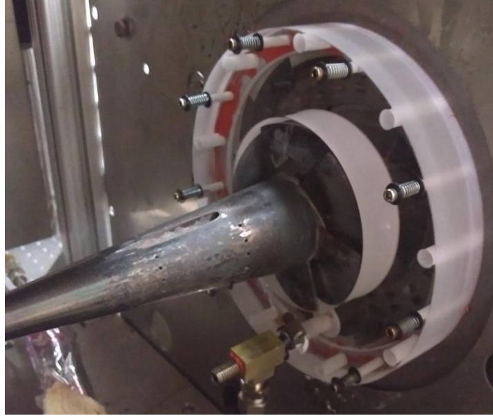
Figure 65: Installed quartz back plate
